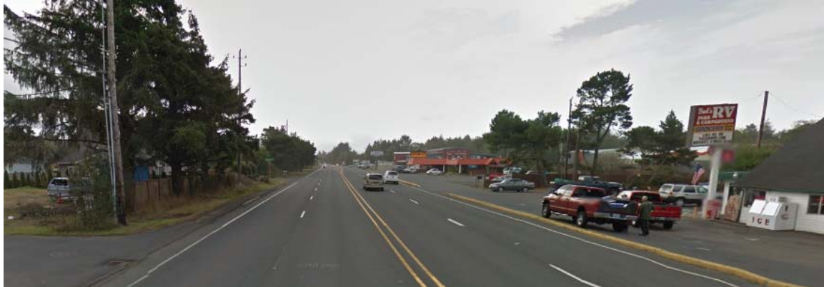
Figure 2-4 – Skinny shoulders with maintenance issues in Gerhart
