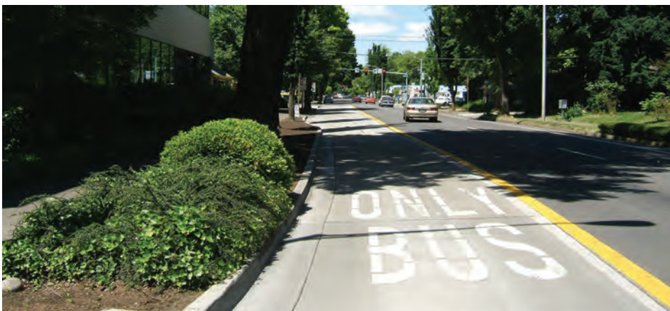
“Bus-only” lanes on LTD’s EmX bus rapid transit system (Photograph credit: CH2M)
